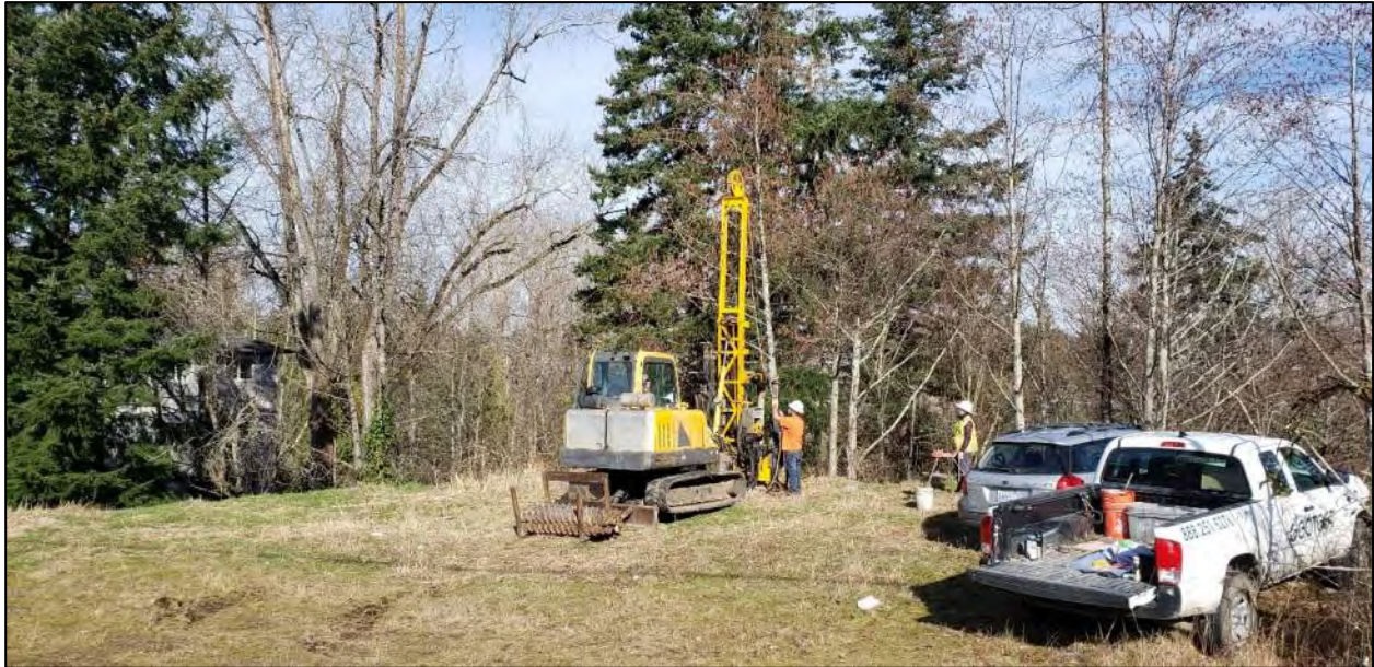
Image 3. Photo of borehole B-1 in progress, facing northwest.
